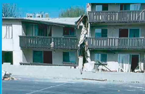
Thousands of buildings like this one are still in use. Many have been reinforced but are still weak and often are not appropriate for living.
