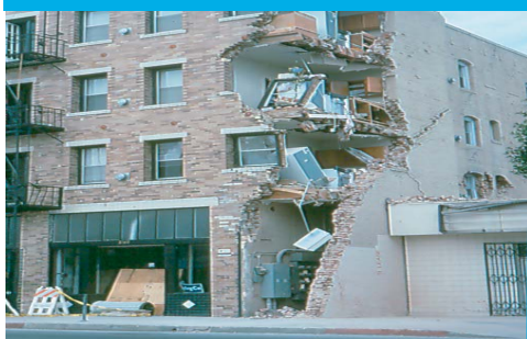
This apartment collapsed due to inadequate lateral bracing. It was too weak to withstand the earthquakes forces.
