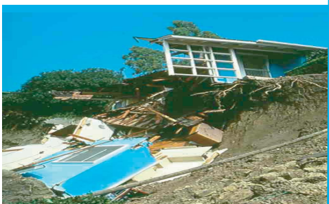
This home completely fell apart when an earthquake caused this landslide. Other houses remained intact even as the landslide pulled out from beneath them.
