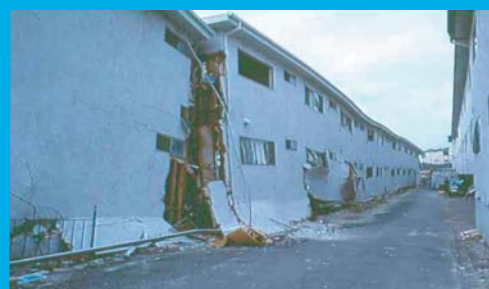
This apartment building had a "soft first floor" causing the first floor to collapse during an intense earthquake.
